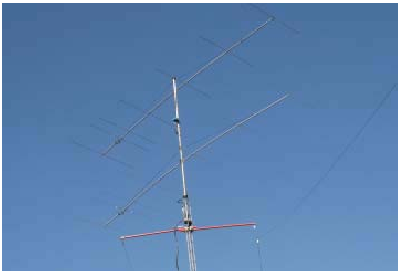
The complete installation on top of the tower.
