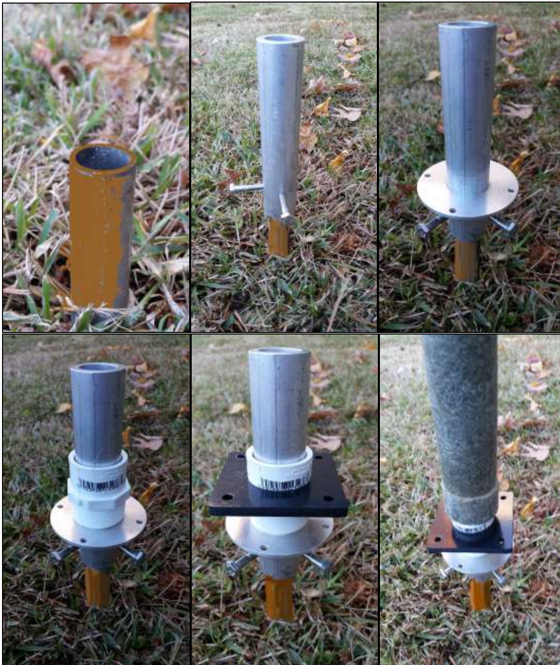
Sequence of base assembly, from the grounding rod to the first mast pipe section
