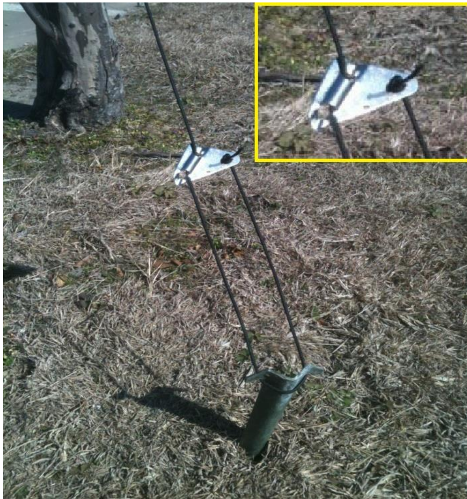
Triangle tensioner installation. See insert for rope threading. Rotate it counter-clock wise for tension release and adjustment.
