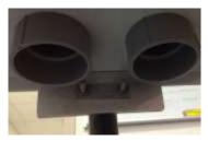
To mount the brackets on your tower (or pipe), remove the two nuts from the Ubolts, and position them on your tower leg at the point where you want the 8-Pak to be placed. Leave the nuts loose enough to separate the two plates a bit to fit the top and bottom flanges of the 8 pak cabinet.
