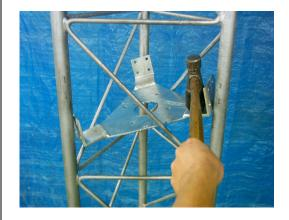
Install and tighten the 6 (six) supplied U-bolts to lock it firmly into place on the tower
