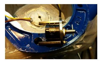
Install the potentiometer in the metal holder and tighten the nut. Put the pin that comes with the potentiometer through its shaft. You may squash the ends of the pin to avoid the pin sliding out of the shaft.
